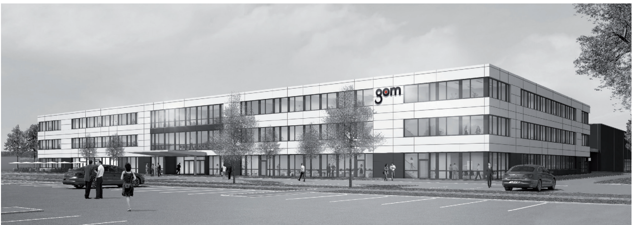
GOM headquarters in Braunschweig, Germany
